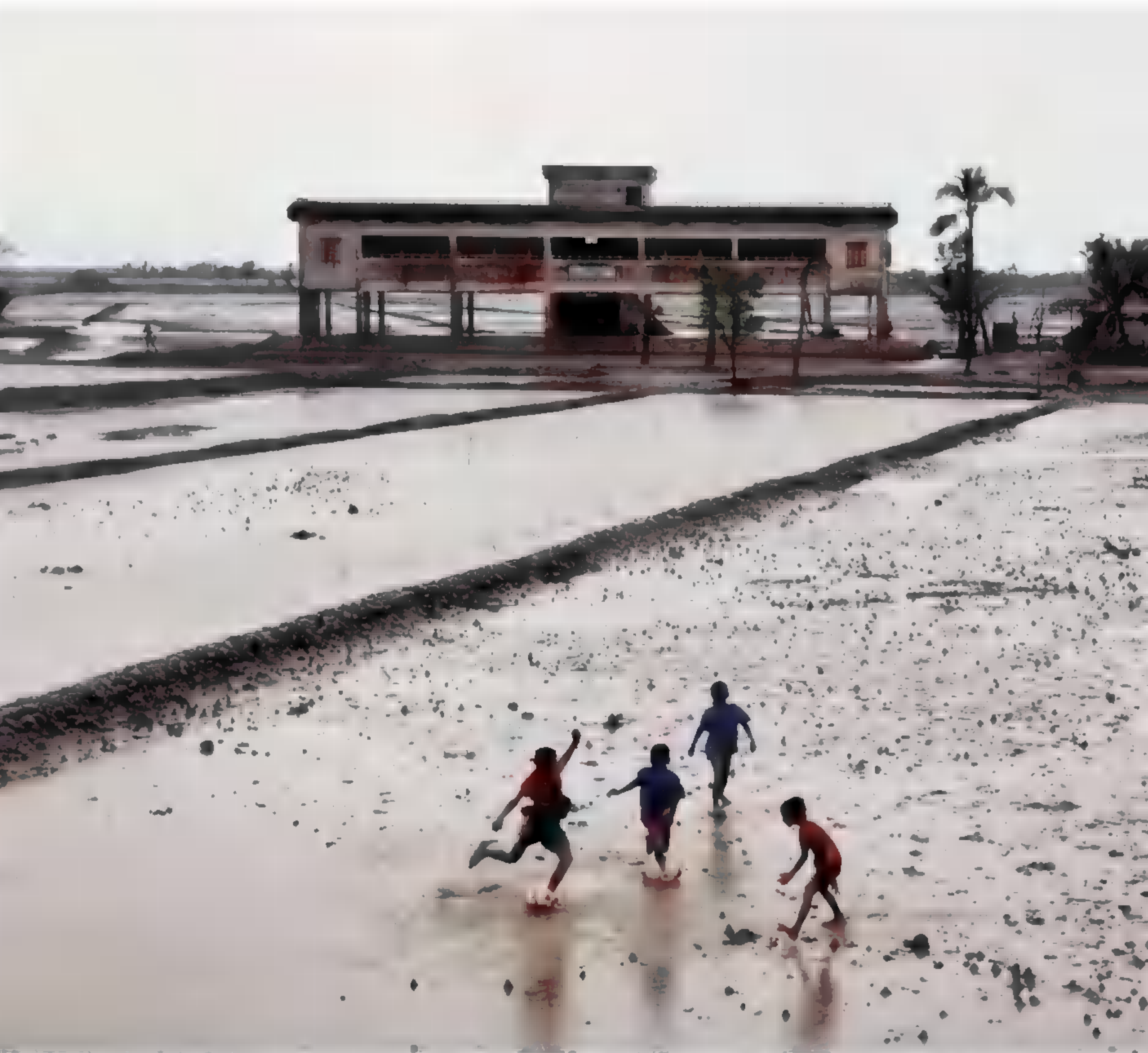
RESILIENT SPIRITS Children play on in Jaliakhali, a village devastated by Cyclone Aila in 2009. That storm sent residents racing for one of thousands of recently built cyclone shelters (above), many of which double as community centers.
